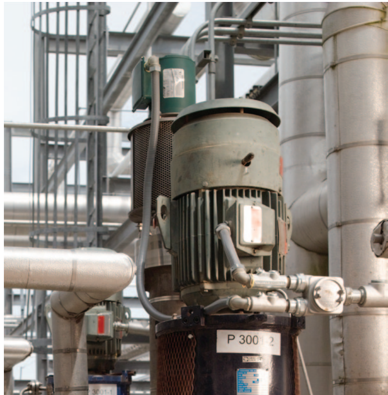
By using thermal imaging, Alltech determined that insufficient airflow and cooling was causing this pump seal to fail, saving a $100,000 project from ongoing seal failure.
