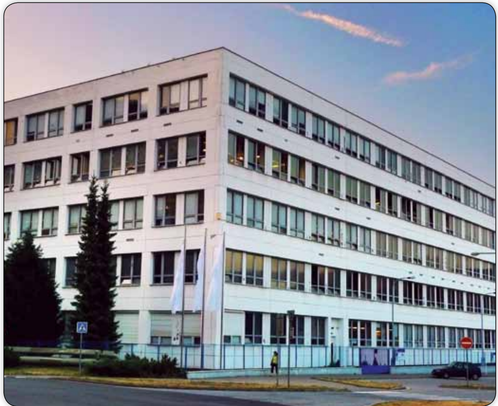
TE Manufacturing Facility in Trutnov, Czech Republic
